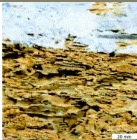
thick layers of limewash on damaged wood
