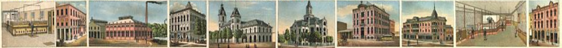
1. THE GREAT CONDOR'S HOME AND BAPTIST HOSPITAL BUILDING 2. W. B. BARTON'S HOME 3. J. J. BROWN'S HOME
