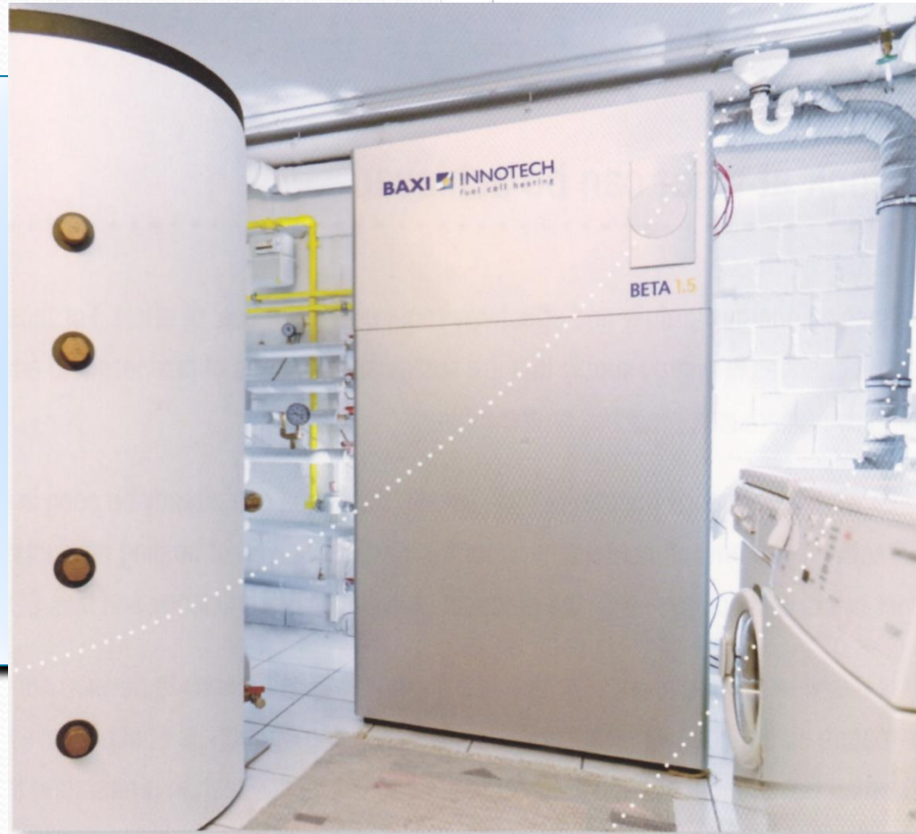
2007: Installation of the BETA 1.5 unit
