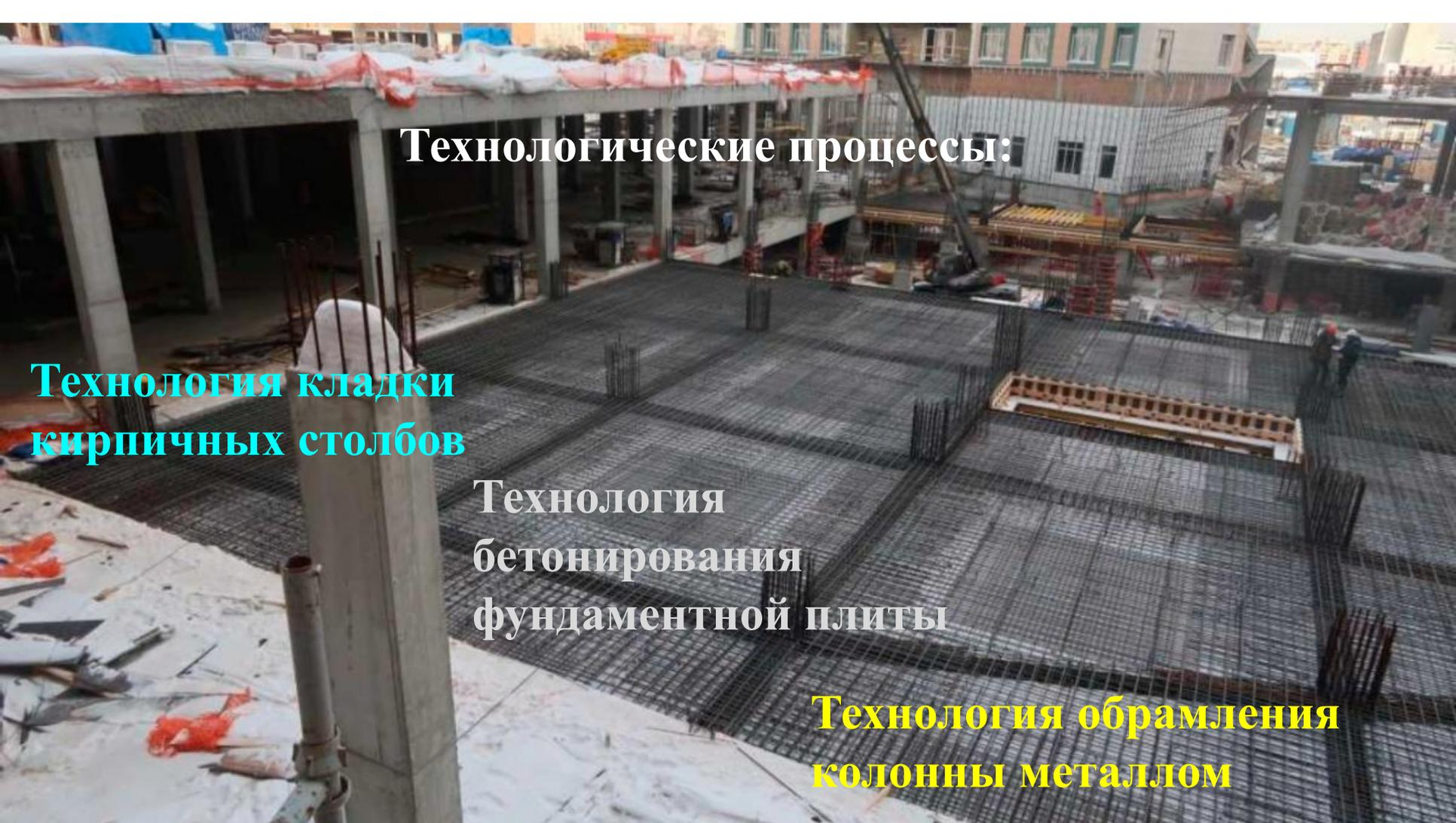
A high-angle photograph of a construction site on a building floor. The floor is covered with a dense grid of steel rebar, prepared for a concrete pour. Several brick columns are visible, some with metal reinforcement. In the background, there are other buildings and construction materials. The scene is active, with various construction elements and workers visible.
