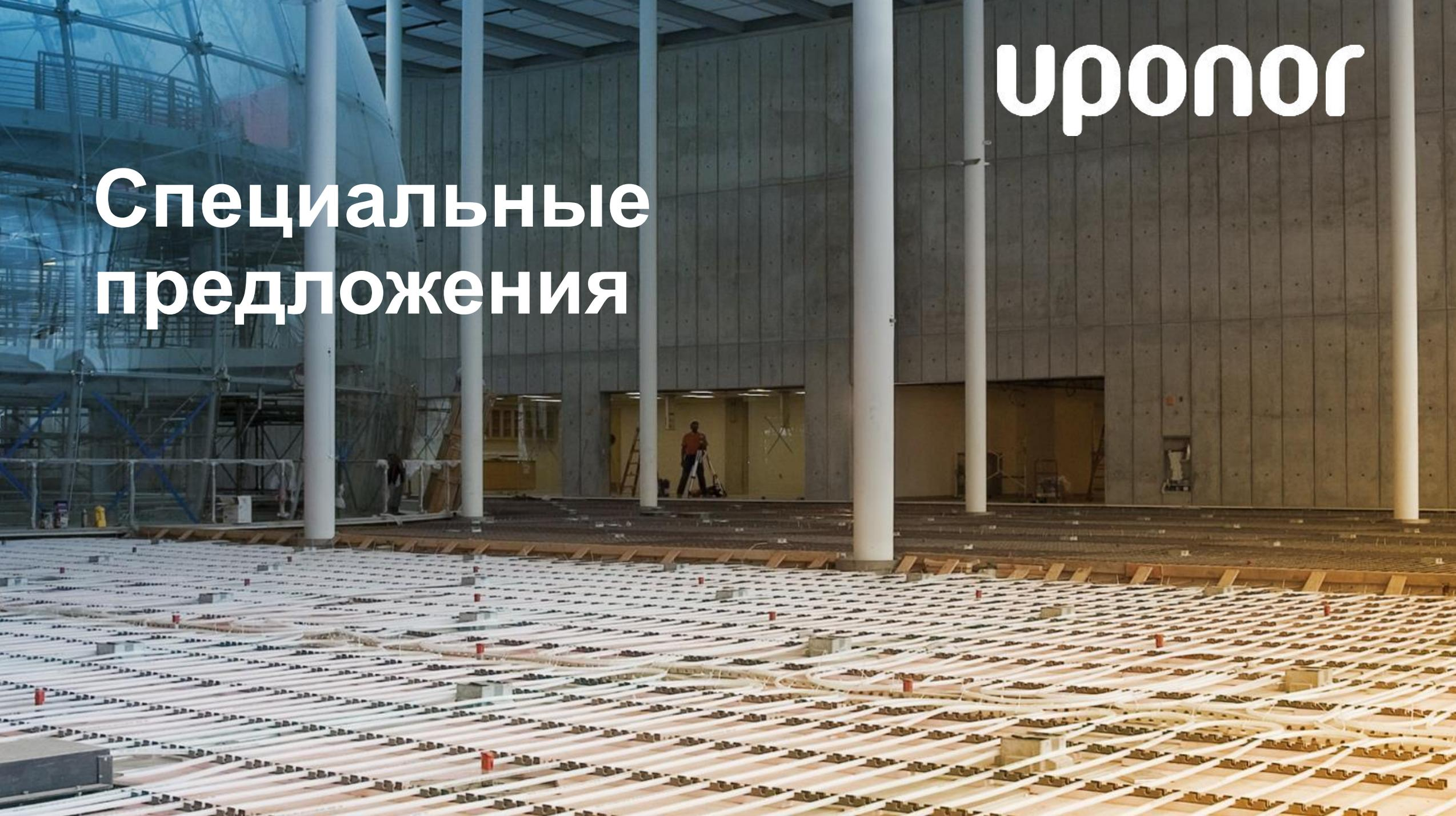
A large-scale construction site interior. The foreground is dominated by a dense grid of steel reinforcement bars (rebar) laid out on a wooden formwork base, prepared for a concrete pour. The background features a massive concrete wall with several tall, slender white columns. A worker in a red shirt is visible in the distance near a doorway. The lighting is a mix of natural light from the left and artificial light from the right.
