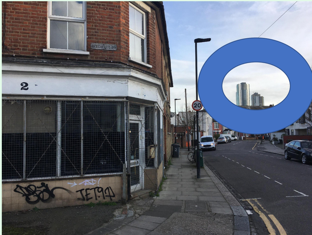
Urban decay in the N4 area
