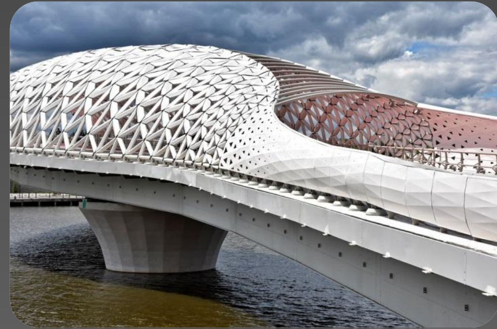
Bridge in Nur-Sultan
