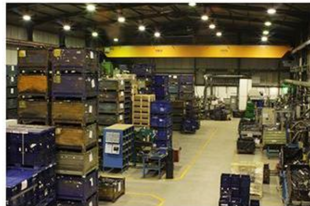
Before (400W High Pressure Sodium)
