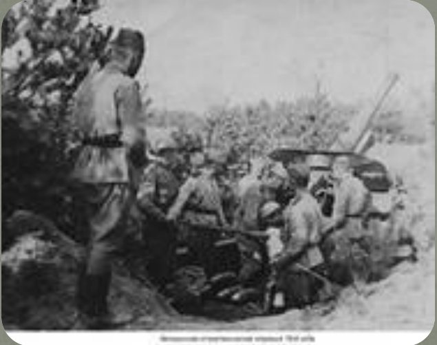
Small, illegible caption text at the bottom of the trench photograph.
