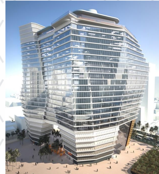
City Gate Tower
