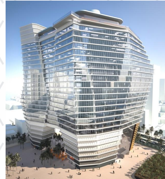
City Gate Tower
