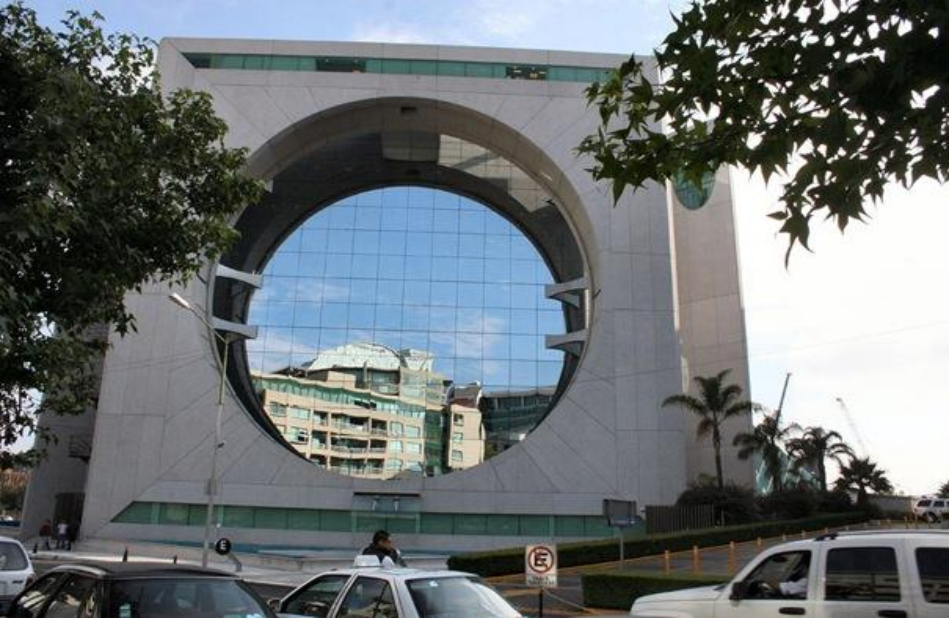
13. Calakmul building a.k.a La Lavadora a.k.a The Washing Mashine (Mexico, Mexico)
