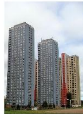
A block of flats
