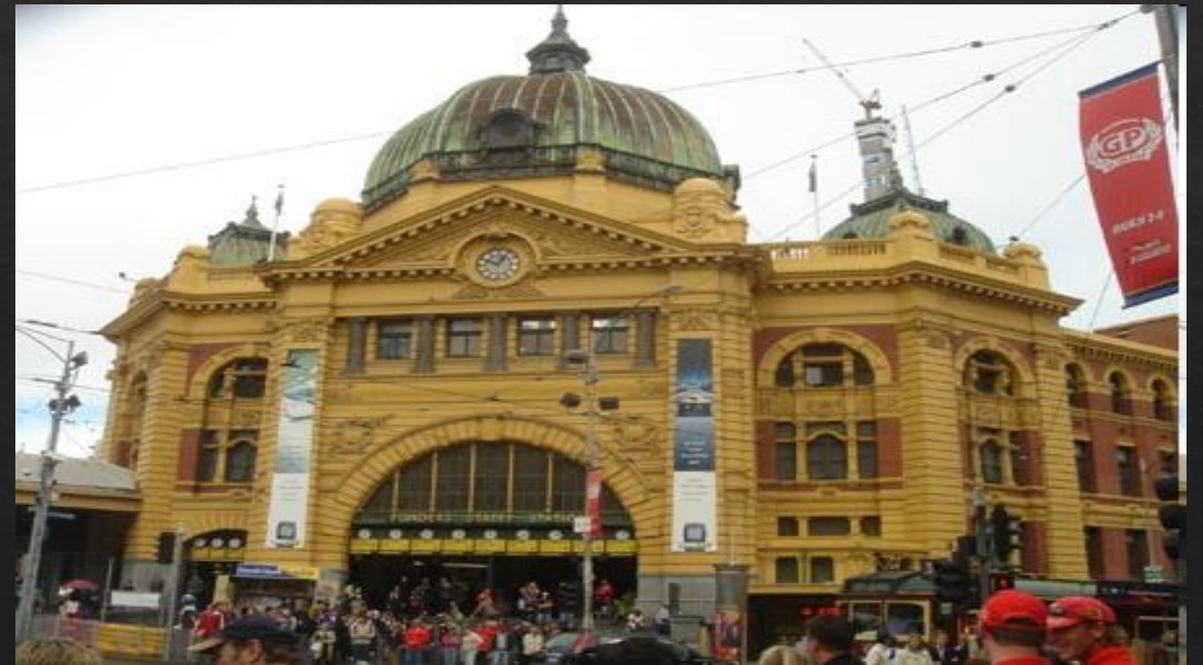
Flinders Street Station
