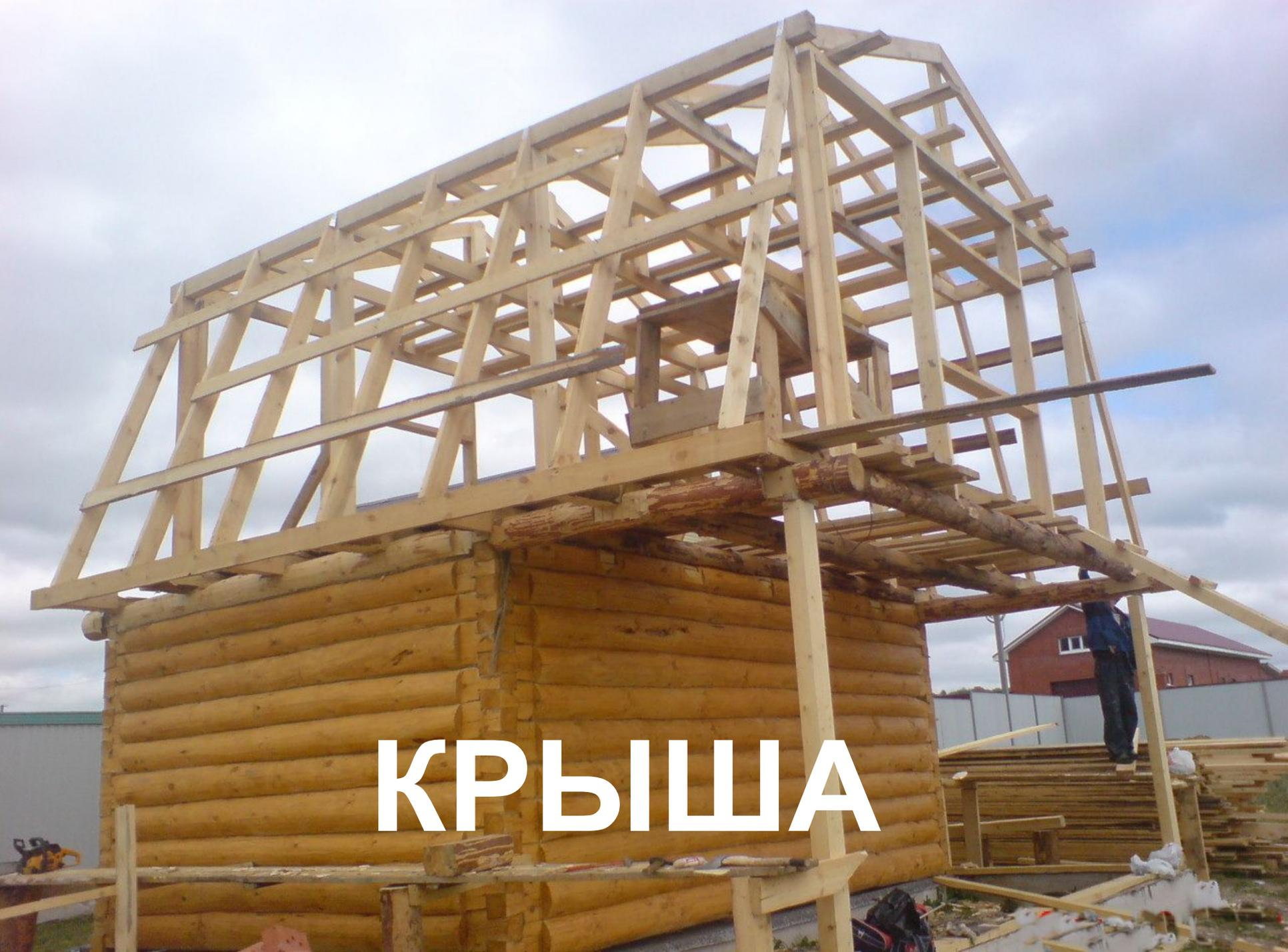
A photograph of a log cabin under construction. The lower portion of the building is made of horizontal log walls. The upper portion is a complex wooden roof structure with numerous rafters and beams. A person in a blue jacket is visible on a wooden platform or scaffolding on the right side of the roof. The sky is overcast and grey. In the background, there is a red building and a grey fence. The word "КРЫША" is written in large white letters across the bottom center of the image.
